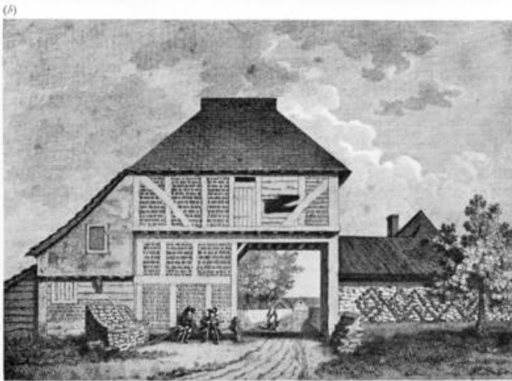
ST. BARTHOLOMEW'S HOSPITAL, SANDWICH (a) CHAPEL (b) GATEWAY
